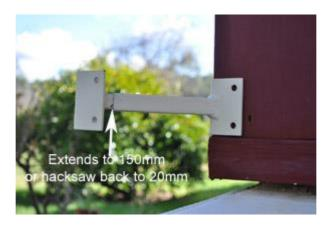
One end of the corner plate is then fastened to the window frame, the other end fixed to the back of the guides, the corner plate is adjustable so it can fit on wall or in reveal fixings, cut the excess of the corner plate of when you have achieved the correct distance out from the window.
