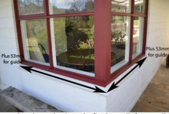
Don't forget to add the 55mm to the other end so it can be fixed on wall (for on wall fixing only). IR (in-reveal) is the same principal, the distance from the window frame must be the same distance on both ends.
