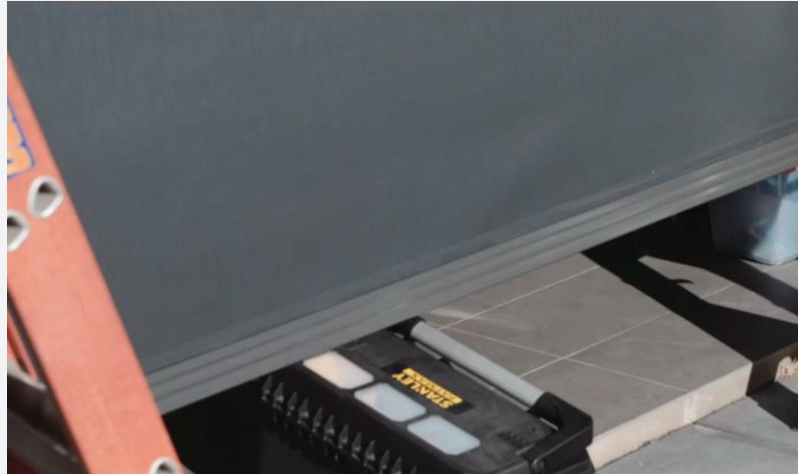
*Picture above of tool box taking the weight of the bottom bar
