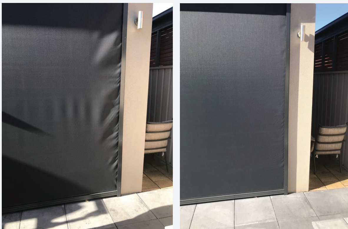
*Picture above: the exact same blind – Left is immediately after install, Right is after 40 minutes in direct morning sunlight.
